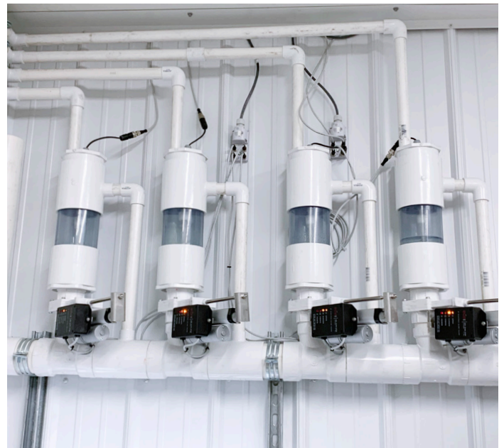
Array of SCS Dehu Meters on Individual Drain Line
