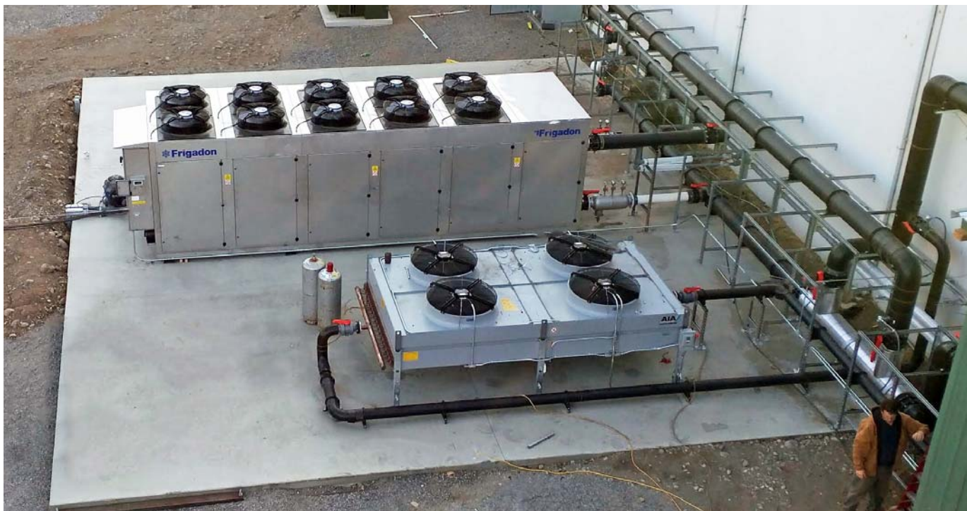
Free Cooler Option using Outdoor Ambient Temperatures for Cooling during Winter Months
