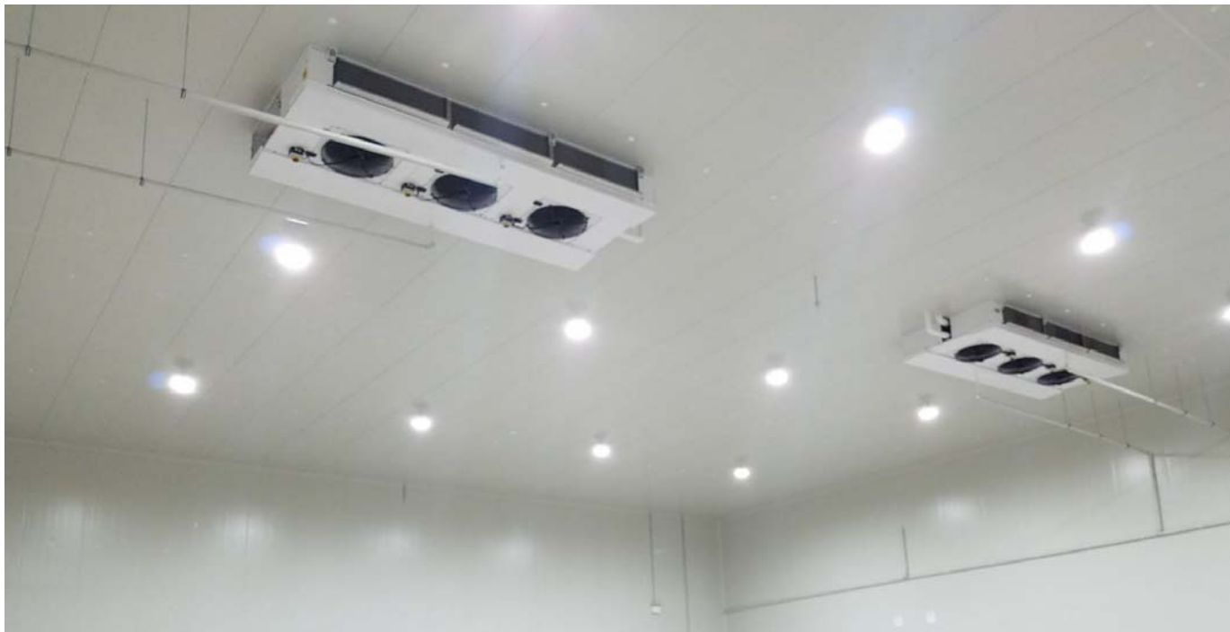
Low Profile Dual-Discharge Refrigeration Coils use Less Space above with Increased Airflow
