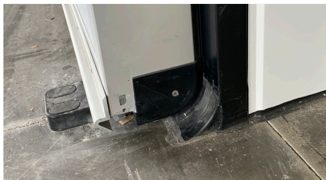
Improved Case Radius at Bottom of Doors for Better Seal
