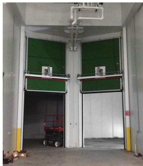
Vertical Lift Gastight CA Door with Motor
