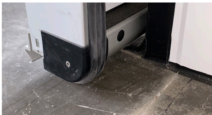
Improved Seal Radius at Bottom of Doors for Better Seal
