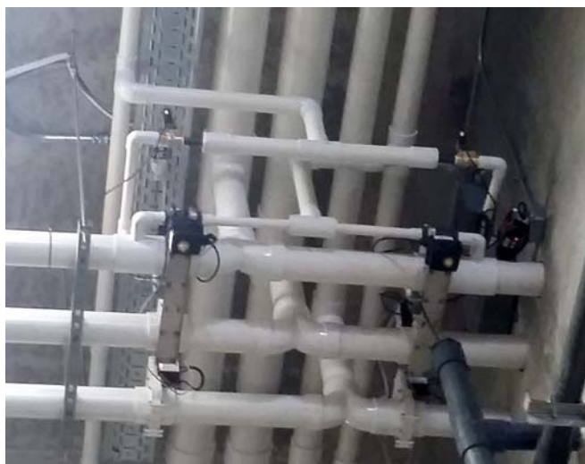
IntelliVent Line (at Far Left) Ducted to Room Scrubber Discharge
