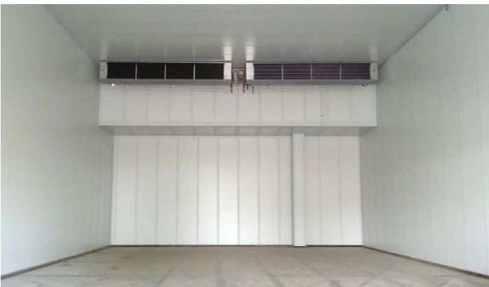
Gastight Sealed Insulated Metal Panel Storages with Secondary Refrigeration Heat Exchangers & Chillers
