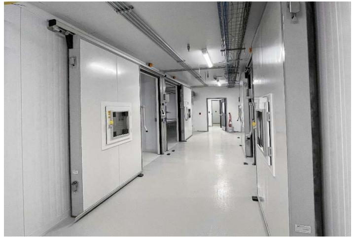
Interior Facility Fit-Out with Secondary Refrigeration Piping & Gastight Room Doors
