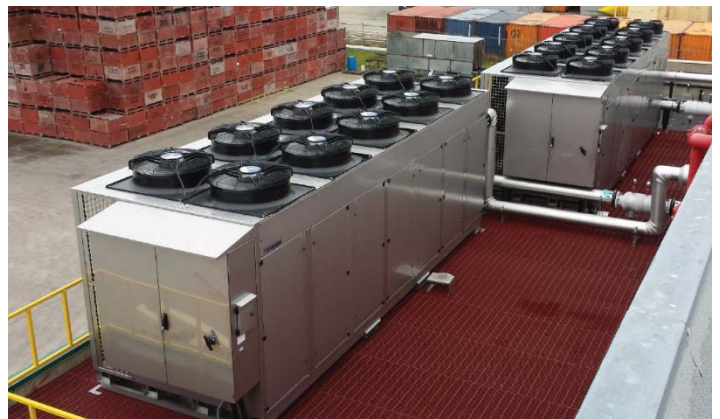
Gastight Sealed Insulated Metal Panel Storages with Secondary Refrigeration Heat Exchangers & Chillers
