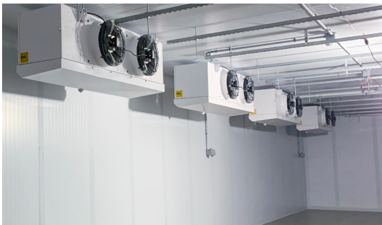
Back-to-Back Coil Arrangement over Aisle in Room
