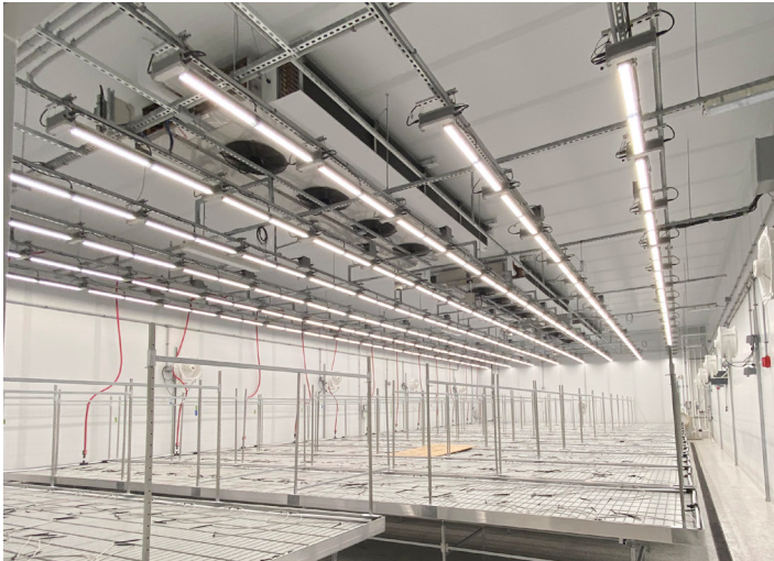
Lights Hang Below Coils for Maximum Canopy Height
