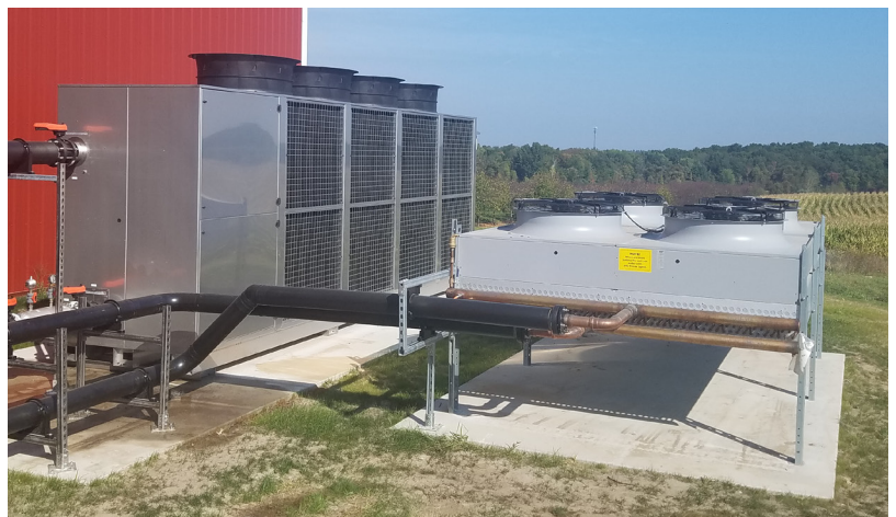
Chiller with Free Cooler Option using Outdoor Temperatures for Cooling
