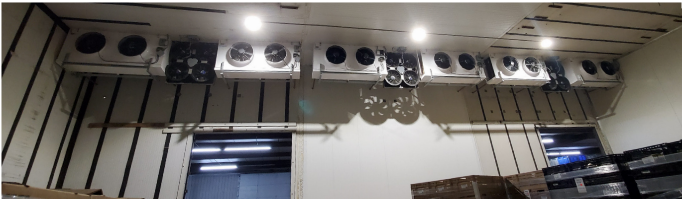
SCS Draw-Through Coil Design Implimented into Existing Onion Storage
